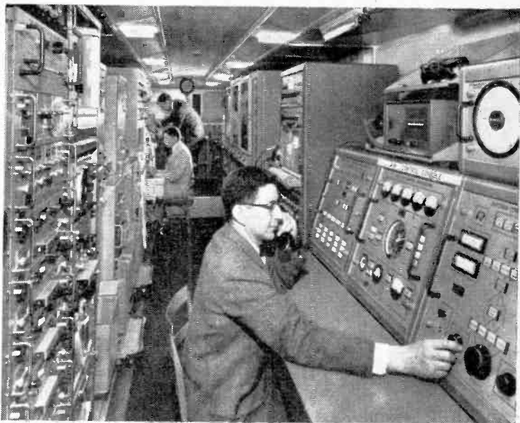
Fig. 2. Control console, klystron recorder and tape machines in the control van for the Courier project.
